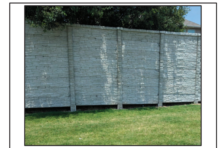
MASONRY SCREEN WALL ABOVE PHOTO OF EXISTING SCREEN WALL WAS TAKEN ALONG THE REAR OF THE TACO BELL SITE WEST OF THE PROPOSED AUTOZONE. PROPOSED SCREEN WALL ON AUTOZONE'S SITE TO MATCH THIS WALL. CONTRACTOR SHALL SUBMIT SHOP DRAWINGS FOR AUTOZONE AND CITY OF LAVON REVIEW AND APPROVAL PRIOR TO MATERIAL ORDERING OR WALL CONSTRUCTION. MANUFACTURER: HANK CONSTRUCTION WEBSITE: WWW.HANKPRECAST.COM PRODUCT: STACK-CRETE, CHISEL PATTERN MOW STRIP: PROVIDE CONTINUOUS CONCRETE MOW STRIP BENEATH WALL PER MANUFACTURER DETAIL AND SPECIFICATIONS (WHOLLY CONTAINED ON AUTOZONE PROPERTY).
