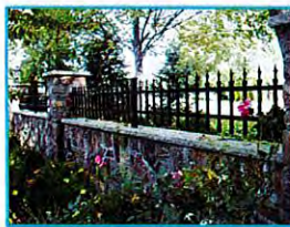
4' HT. MASONRY WALL WITH 2' TUBULAR STEEL FENCE
