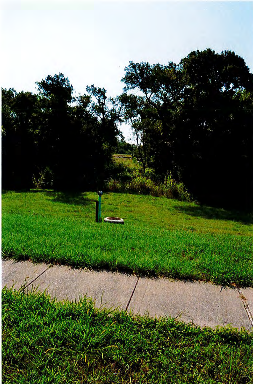
Point of Creek Crossing from the west side of the creek and current connector for Eagle Pond Park and NeSmith Elementary School
