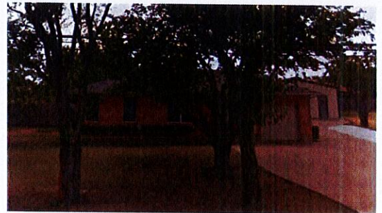
RESIDENTIAL BUILDING – SOUTH SIDE
