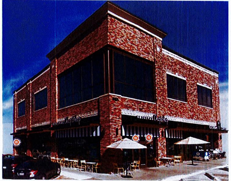
TWO STORY W/ ROOF TOP
