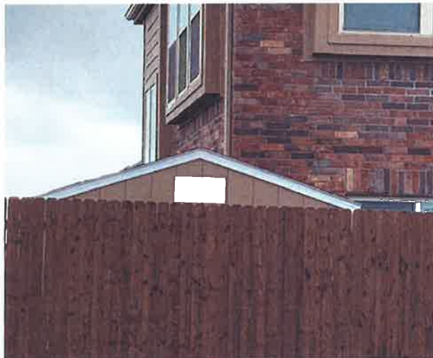
Similar structures - provided by applicant
