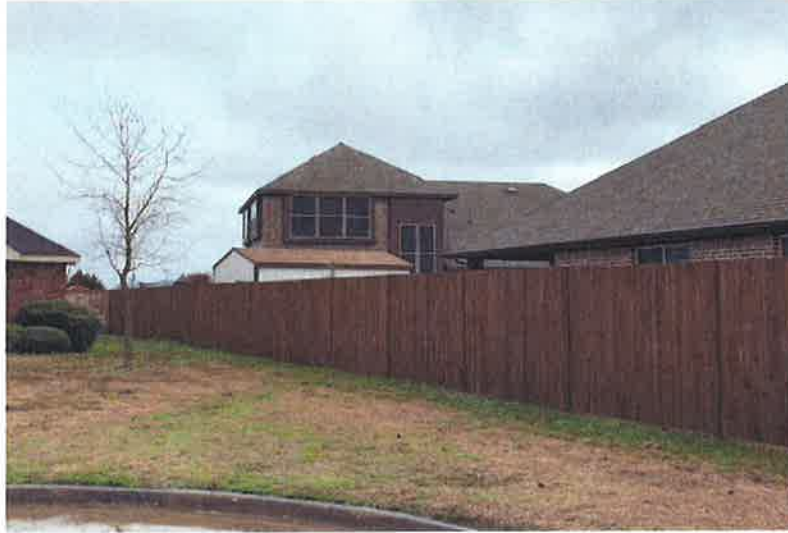
Similar structures - provided by applicant
